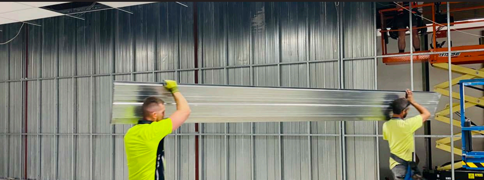
K8 SUPAPANEL® onsite install
